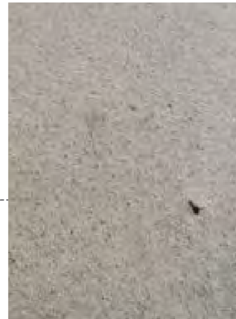
Compacted Gravel fines
