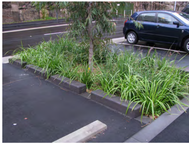
Rain gardenbeds in parking
