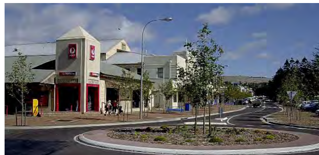
Port Lincoln Town Centre, South Australia
